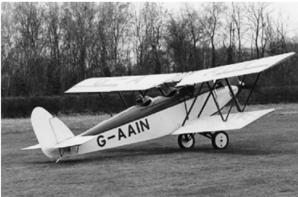
and flying wires inboard of those struts, a system of Warren girders provides the necessary rigidity and even eliminates the need for a jury strut when the wings are folded. The makers' booklet claims that in this condition the Elf is 1ft 6in narrower than other existing machines, to facilitate transport through gateways when being retrieved after a forced landing. How they must have known what was to come!
