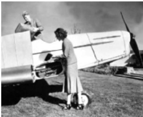
**Above: right wing root held either extra fuel tank or baggage compartment**
