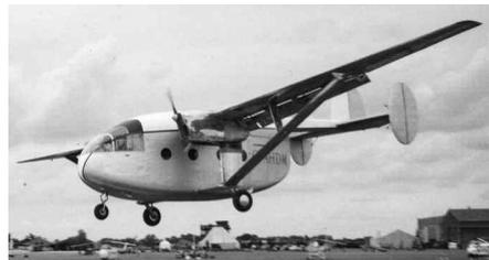
**Above: G-AHDM was fitted experimentally with a very high aspect ratio wing of 75ft span designed by Hurel-Dubois of Villacoublay in France**
